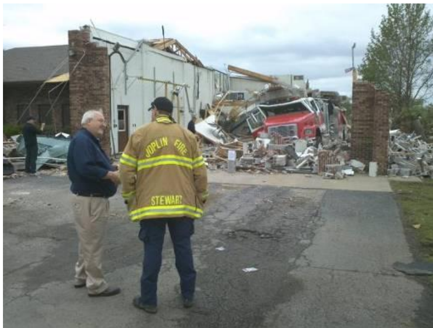
Figure 5: FEMA Administrator Craig Fugate surveys a damaged fire station with a Joplin firefighter. (Source: FEMA)
