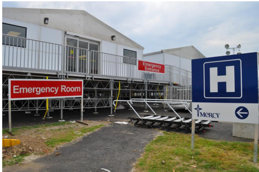
Figure 9: St. John's Regional Medical Center modular hospital units. (Source: FEMA)
