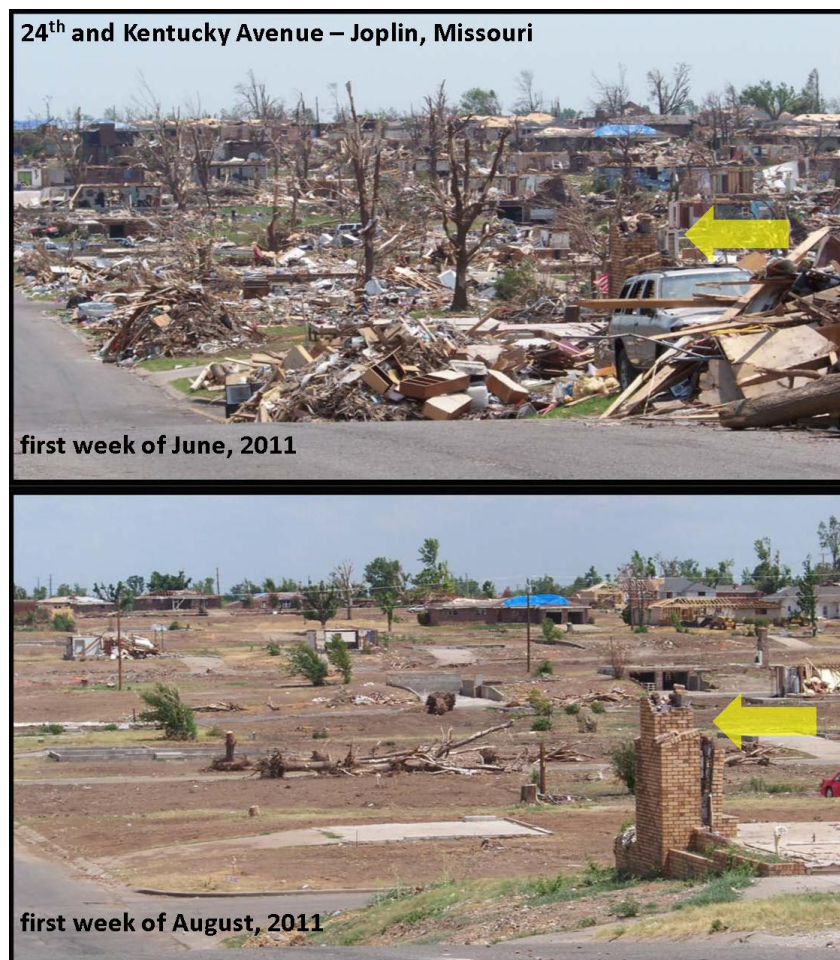
Figure 13: The impact of EDR on a Joplin intersection. (Source: FEMA)
