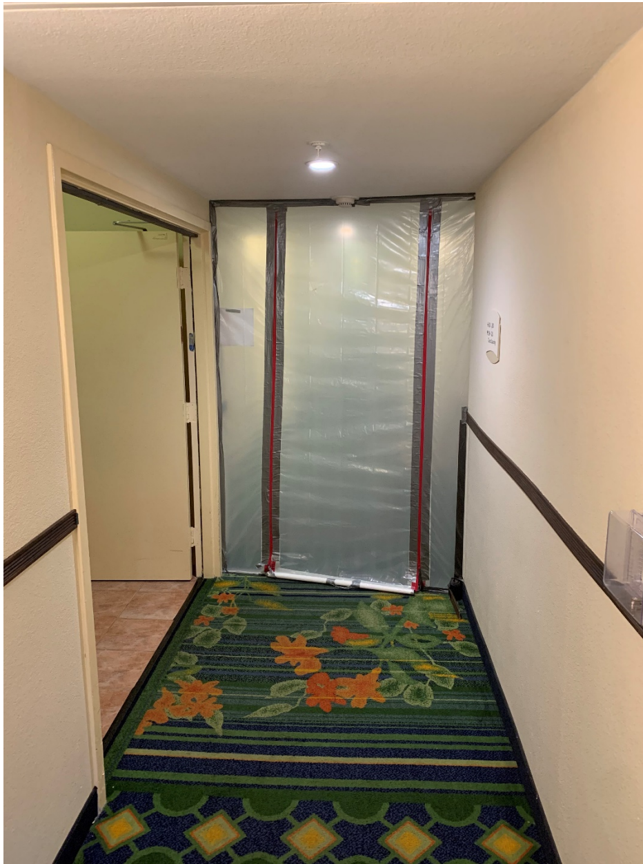
Figure 3: Sample Plastic Barrier to Isolation Zone Area
