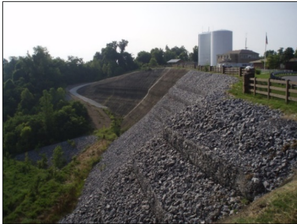
Figure 2-7. Slope stabilization project in Hickman, Ky. (left), and generations of steel piles stabilizing a road in Kenton County, Ky. (right).
