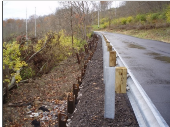
Figure 2-7. Slope stabilization project in Hickman, Ky. (left), and generations of steel piles stabilizing a road in Kenton County, Ky. (right).
